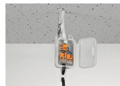
Pendant light connection in a suspended ceiling
