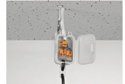
Pendant light connection in a suspended ceiling
